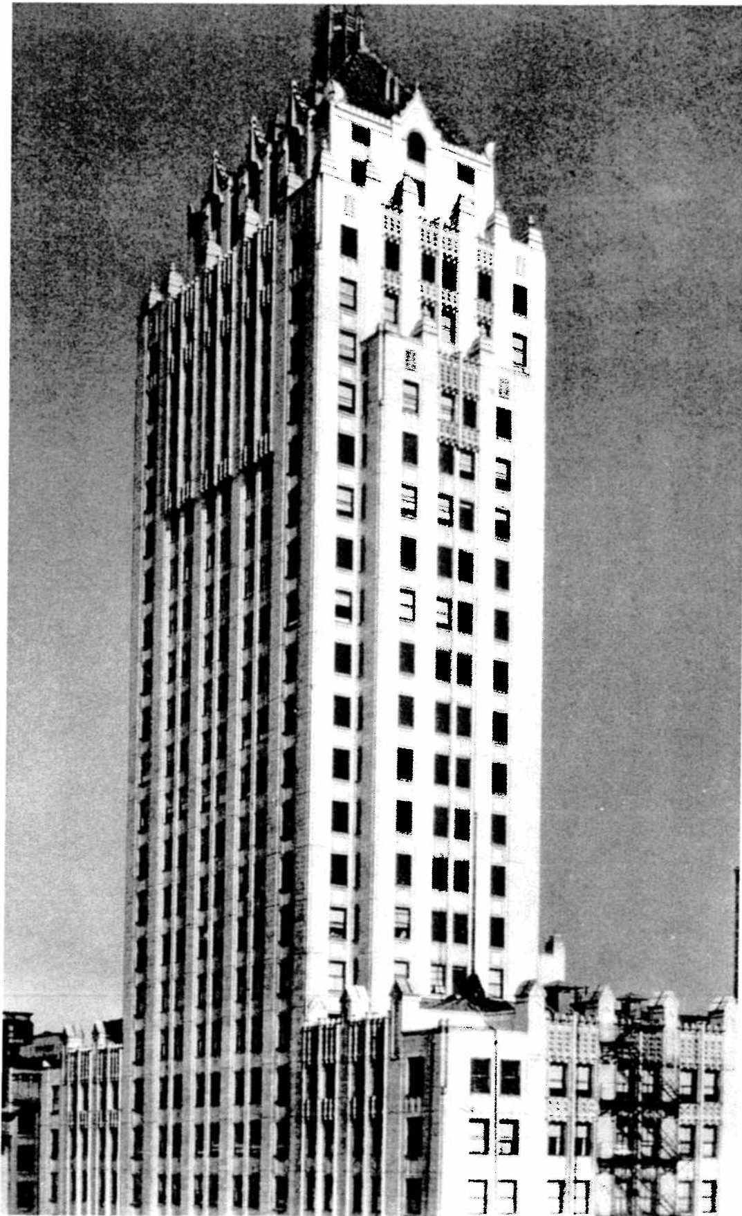
The Pittsfield Building's tower is one of Chicago's most distinctive with its multi-gabled top floor and pyramidal roof of bright green copper.
